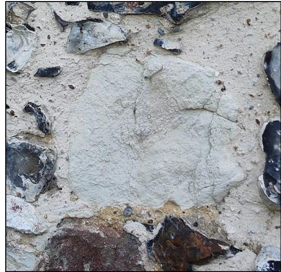
Figure 17: Reigate Stone in north wall.
