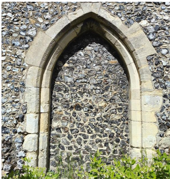
Figure 13: Blocked arch in south wall.
