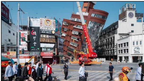
The red brick Uranus building is seen leaning precariously (Credit: Reuters)
