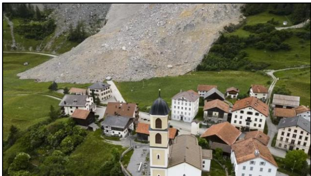
The overnight rockfall just missed the village, coming to a halt close to the local school (IMAGE SOURCE, MICHAEL BUHOLZER /EPA-EFE/REX/SHUTTERSTOCK)
