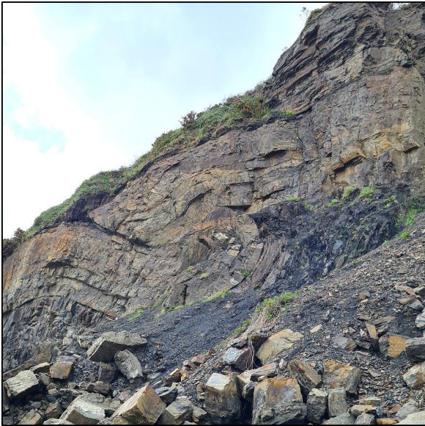
Figure 6: Reverse faults and faulted 'S' shaped folds.
