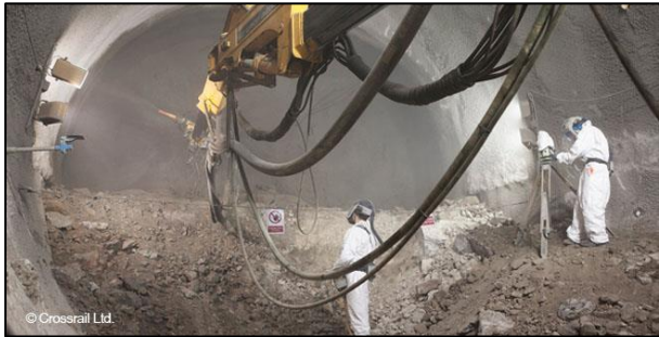
Figure 7: Sprayed concrete lining. (Image: Crossrail Ltd.)
