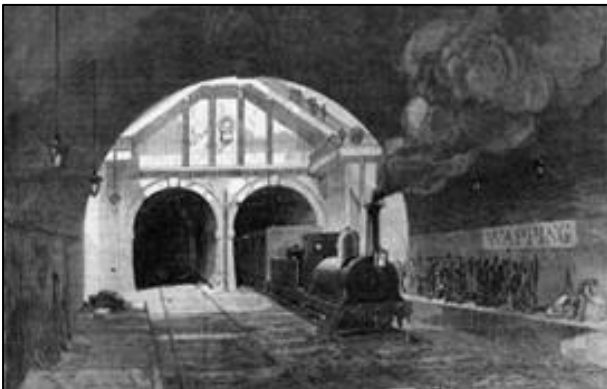
Figure 4: Locomotive exiting the Thames Tunnel and arriving at Wapping station in 1870. (Image: mylondon.news)
