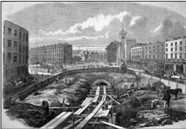
Figure 3: Cut and cover near Kings Cross. (Image: open.edu)
