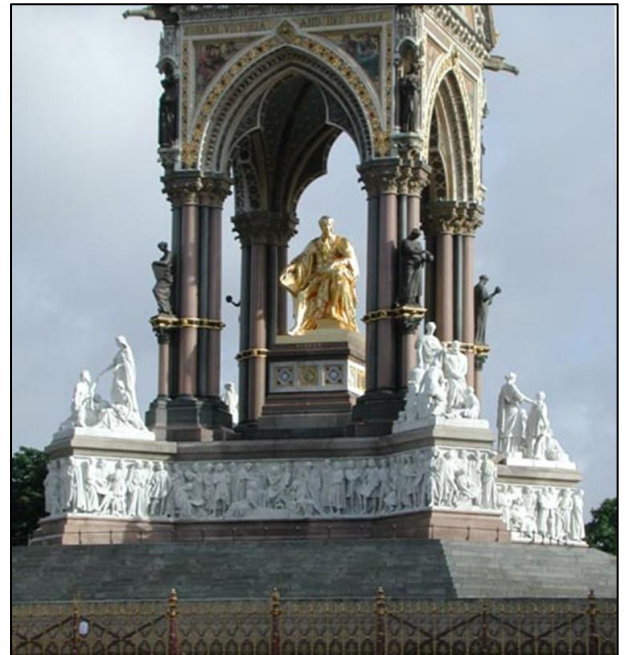
Figure 5: The Albert Memorial designed by George Gilbert Scott in 1863-72. Pink granite from Correnac, Aberdeen, appears with marble in the pedestal on which the statue of Albert sits, while Darley Dale sandstone from Derbyshire is used for the main capitals. The arches are of Portland Stone, while the pillars supporting the canopy are of red granite from the Ross of Mull and a grey granite from Castle Wellan Quarries, Northern Ireland.
