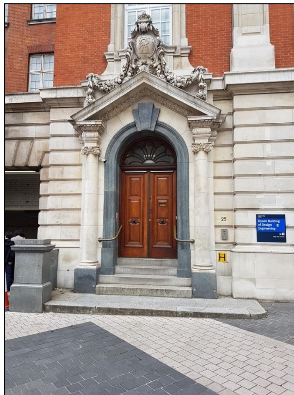
Figure 2: The Dyson School of Design Engineering (former Post Office) building illustrating contrasting granites: (a) dark grey door surround: Aberdeen Rubislaw granite; (b) the steps: Cornish granite; (c) the pavement: Chinese granite.
