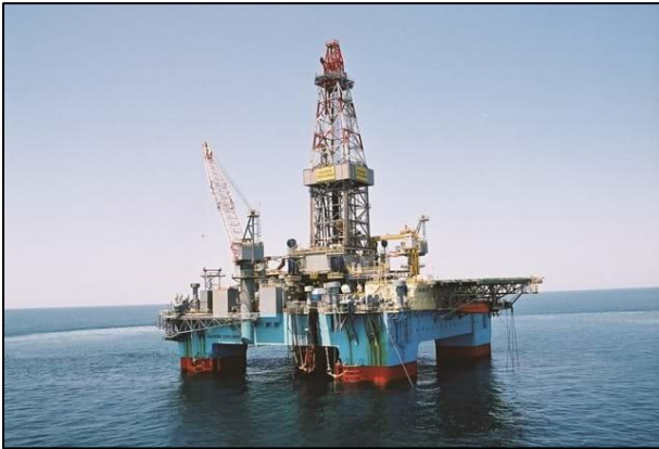
Figure 7: Maersk Explorer Semi-submersible drilling rig. (Credit: Maersk Drilling)
