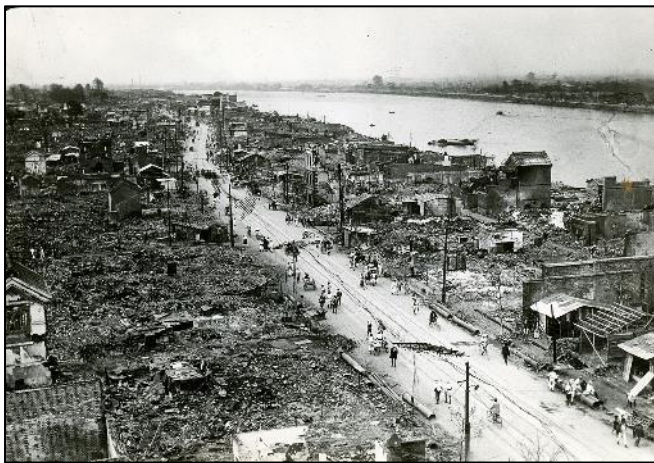
Damage caused by the Tokyo-Yokohama earthquake, 1923. (Image: Encyclopædia Britannica, Inc.)
