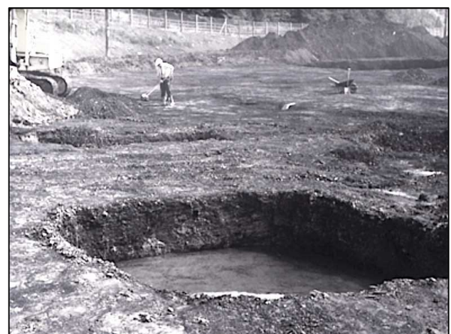
Fig 6: Coal seams previously mined using bell pits.
