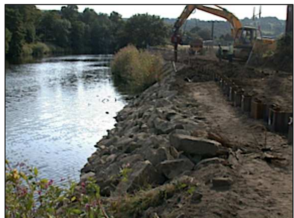
Fig. 15: Sheet pile wall and interception trench, constructed to protect Calder River
