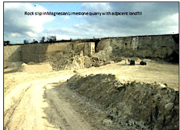
Fig. 12: Moving block of Magnesian Limestone
