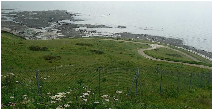
Fig. 32: Holbeck Hall slip of 1993, now landscaped.
