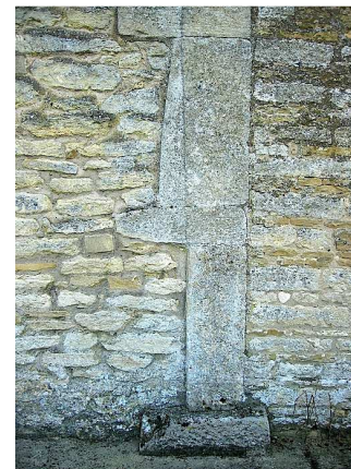
Fig. 6: The NE chancel quoin, Wittering Church (Peterborough) has quoins cut back so all stones look of equal width.
