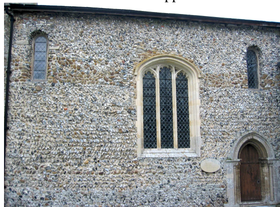
Fig. 7: Hadstock Church in Essex possesses double-splayed windows & remnants of horiz. colour banding in brown Bunter cobbles.
