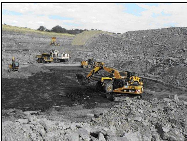
Figure 1: The large 'digger' at the back removes the bulk of the spoil, the small digger in front scrapes off the last layer exposing the coal bed for mining
