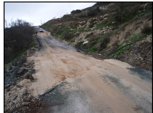
Photo 2 – Landslide affecting new road.
