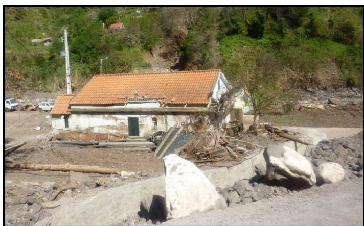
Fig. 5. House and road inundated by debris
