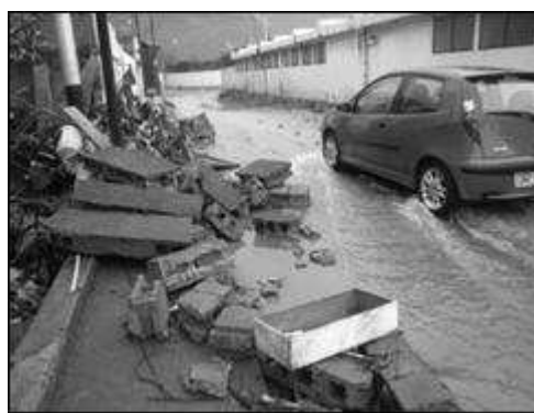
Flood damage to buildings and roads still flooded
