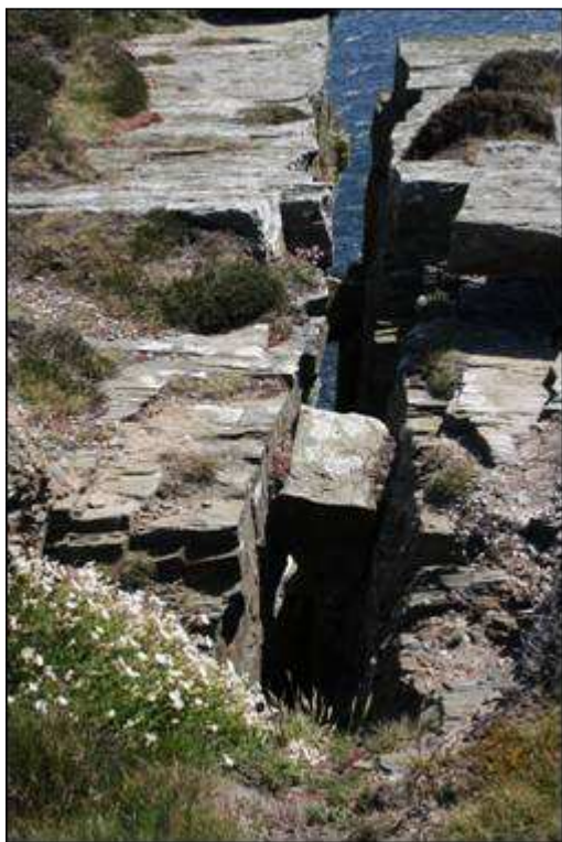
Fig 2: Mega-cracks in quartzite
