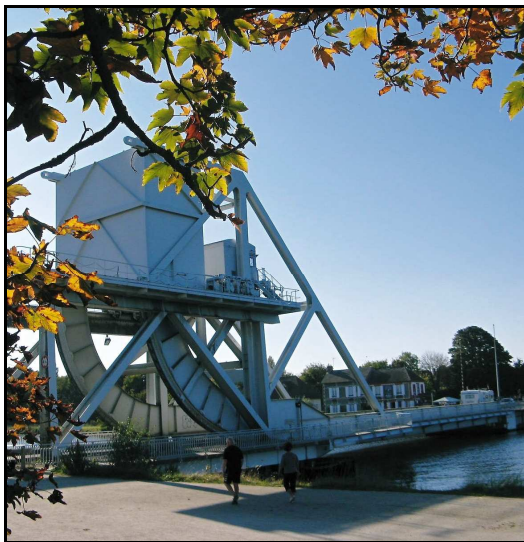
Fig 3: The replacement Pegasus Bridge over the Orne canal
