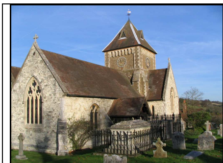
Fig. 5 - Upper Greensand Seale parish church
