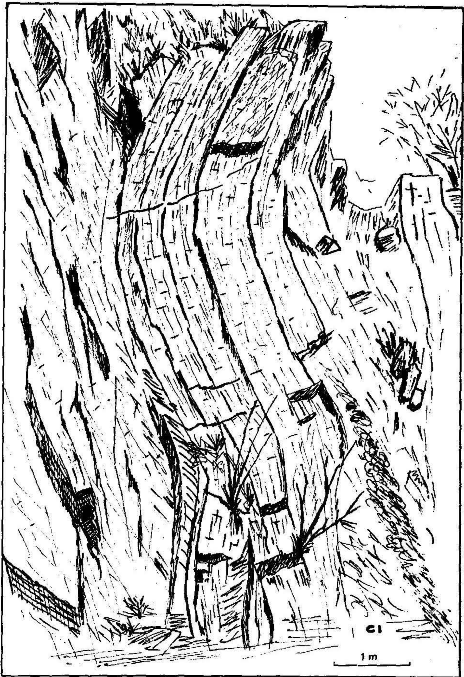
FIG. 2 Gravity slumping in near vertical K-zone Carboniferous Limestone Cement Works Quarry, Mitcheldean, Gloucs. (SO 659183).
